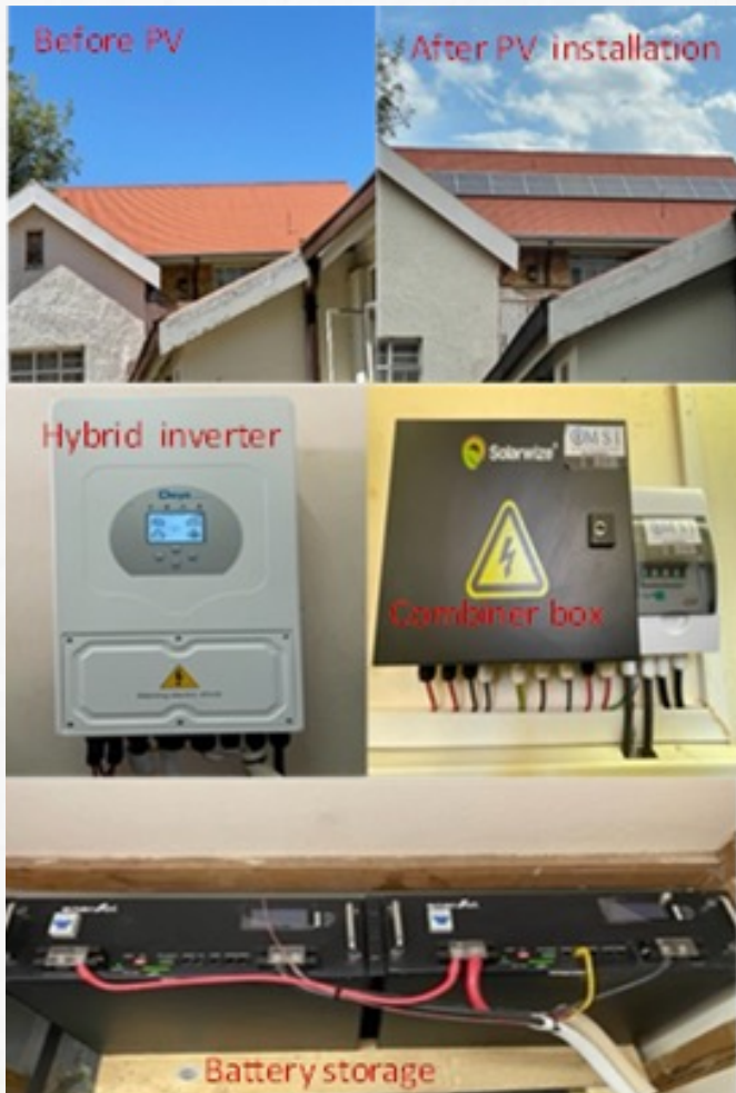
The residence's roof before and after PV installation and the major solar components of the hybrid PV system with battery backup.
